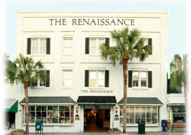
Figure 8: Renaissance Building, 42 ft. (1922)
